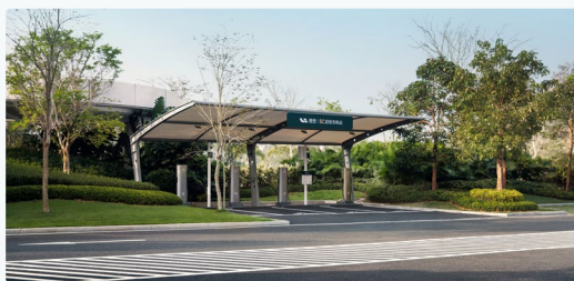
Charging network construction projects
