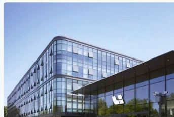
New construction, renovation, and expansion projects for workplace research and development
